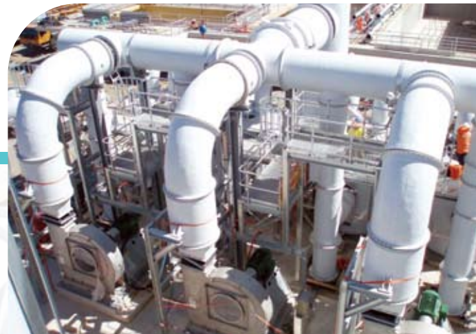
Murrumba WWTP, Australia
